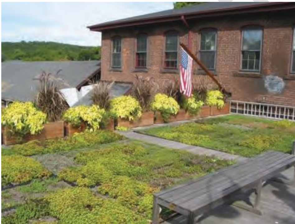
Figure 4.20. Green roof (photo: Center for Watershed Protection, Inc.)
