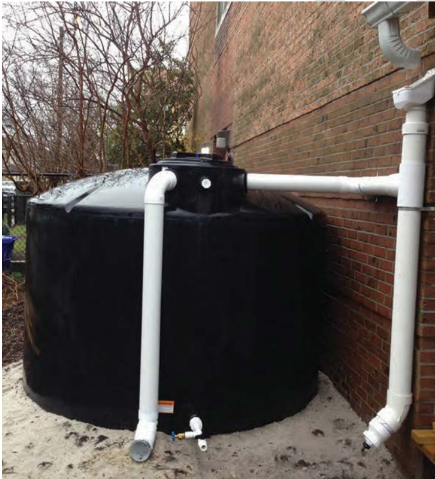
Figure 4.23. Example cistern application (photo: Marty Morganello).
