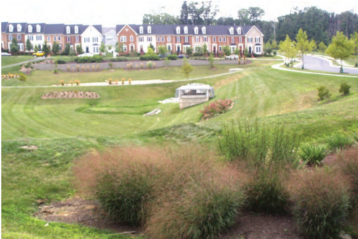
Figure 4.47. Dry Extended Detention Pond (Photo: Center for Watershed Protection, Inc.)
